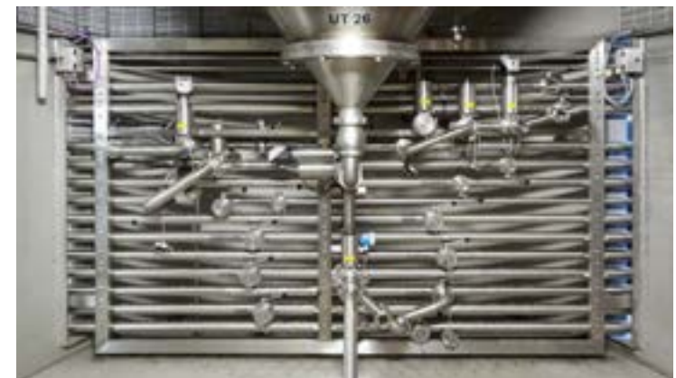
Pipe fence semi-automated
