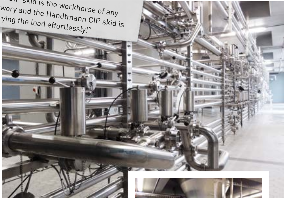
Upgraded and extended pipe fence in 2017
