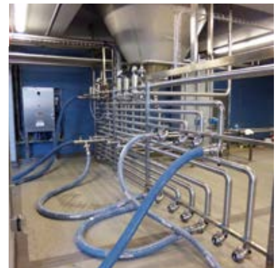
Pipe fence for start up with hoses in 2015
